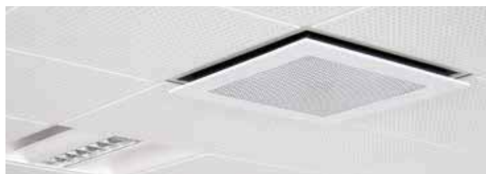
PLM - Metal ceiling panelling with Coanda effect.
